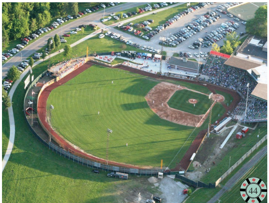
Phil Welsh Stadium Renovations
