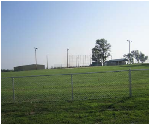
Ballpark Repairs including New Lighting, Fencing, Bathrooms & Concession Stand
