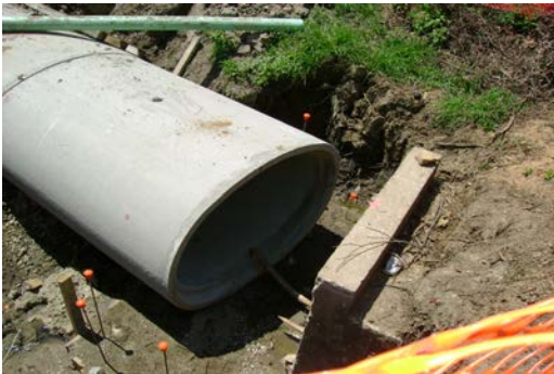
Bee-Jay Drive Storm Sewer Project
