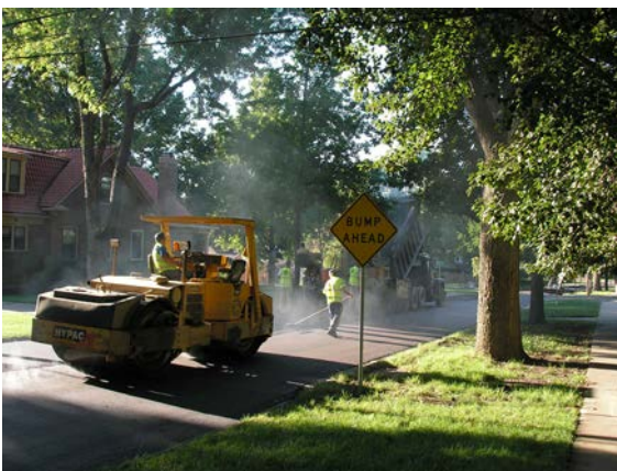
Repaving Roads throughout the City
