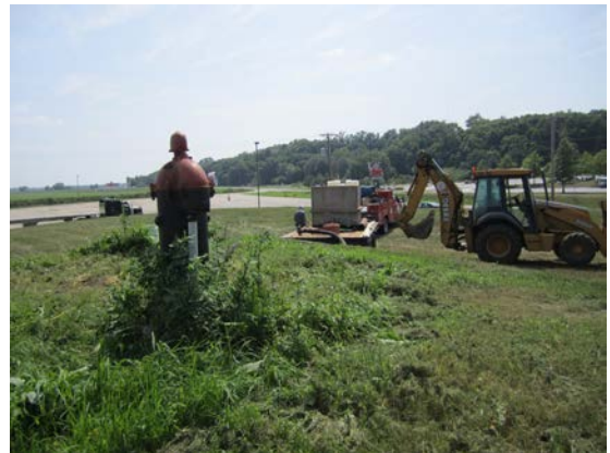
Work on Water Wells
