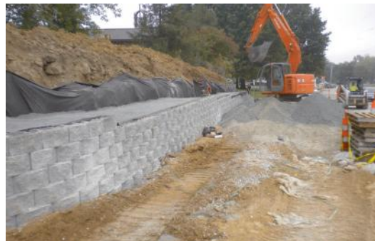
Retaining Wall at Muegge Road
