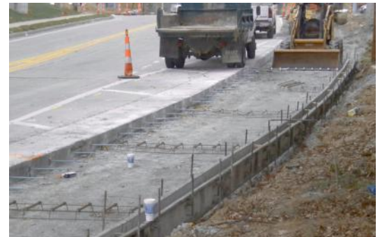
Pavement Subgrade Preparation
