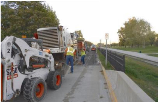
Asphalt Overlay on Riverside Drive
