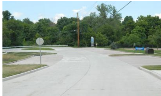
Construction of McKelvey Woods Court
