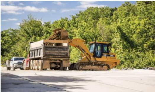
McKelvey Woods Construction
