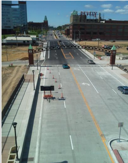
New Grand Avenue Viaduct
