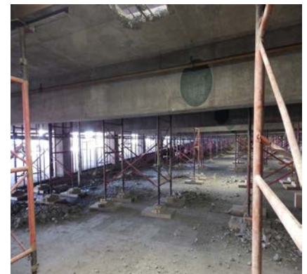
Structural Garage Improvements
