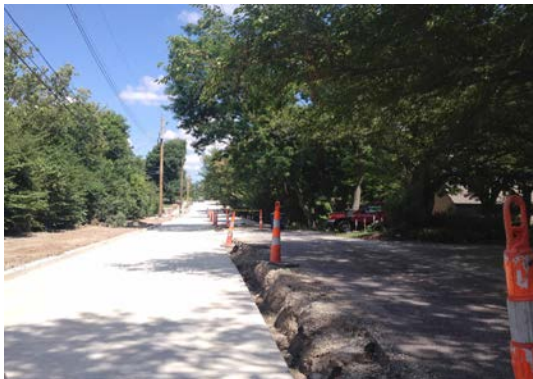
Driftwood Lane Improvements
