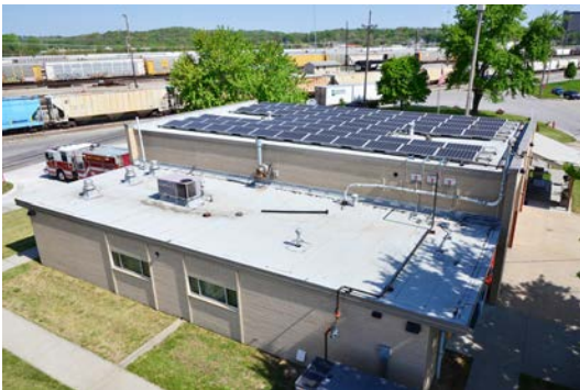
Solar Array on Fire Station
