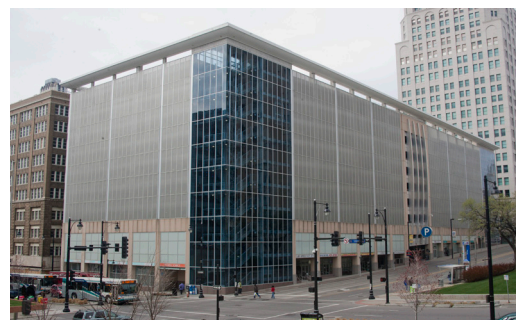
Wolf Parking Garage
