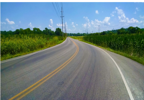
Creve Coeur Mill Road Resurfacing
