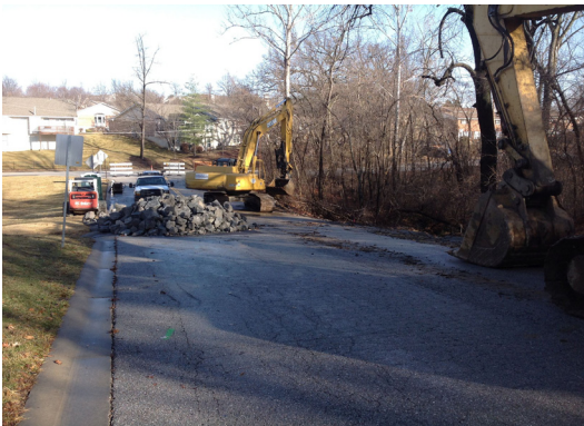
Rio Vista - South 5th Street Culvert Replacement
