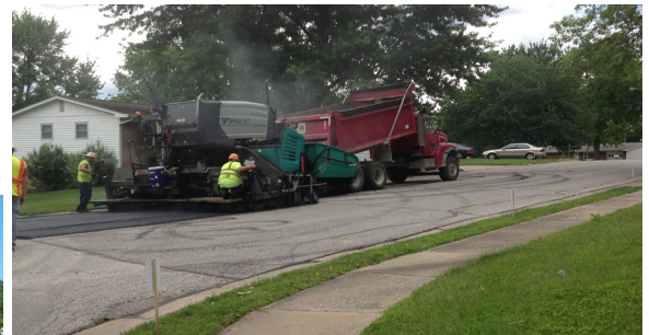
Asphalt Street Repair
