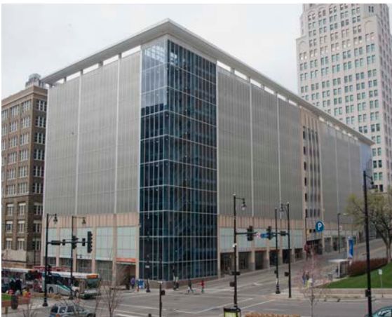
Wolf Parking Garage
