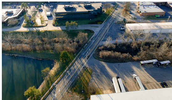
Road and Bridge Work
