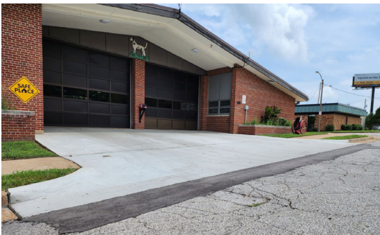
Fire Engine House
